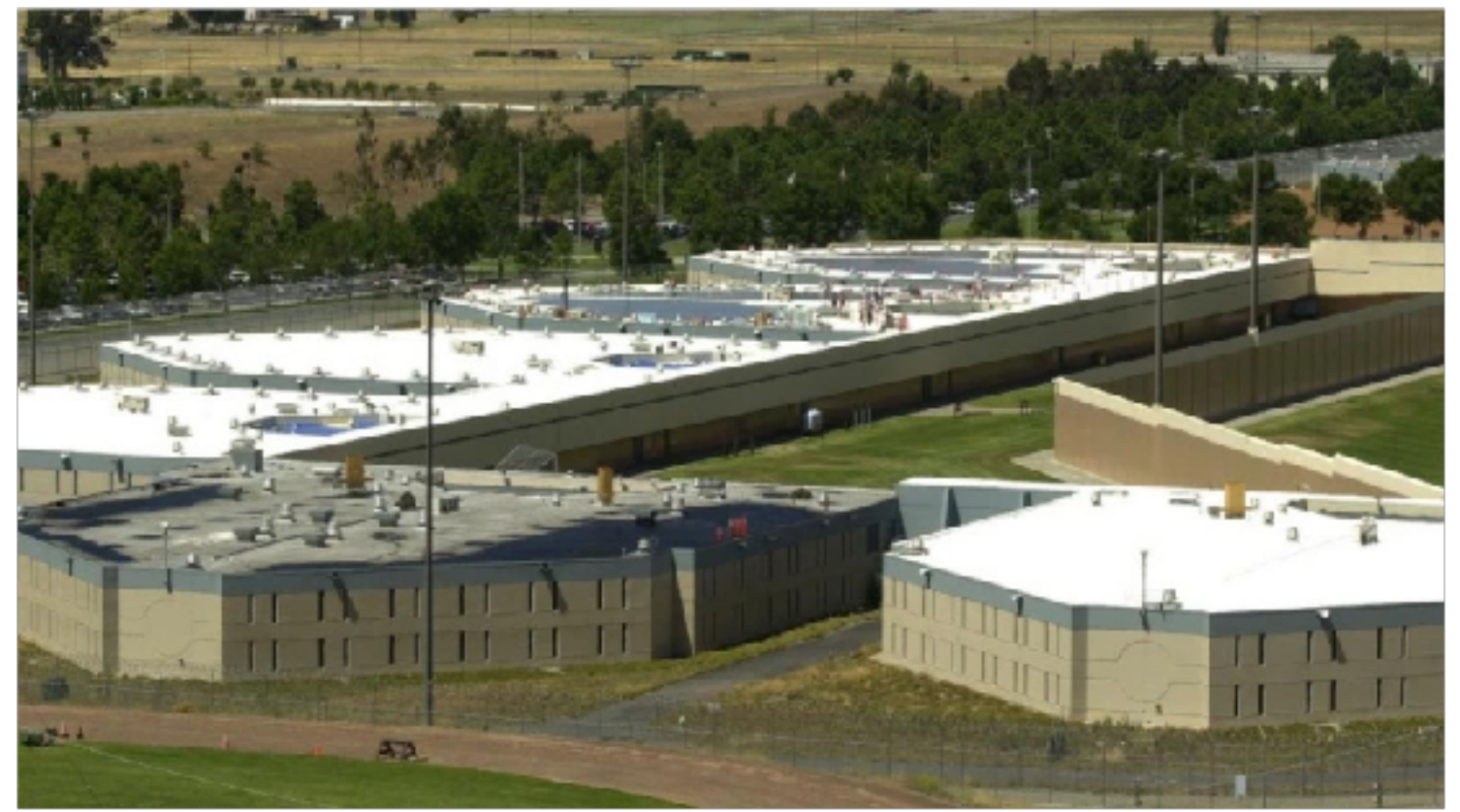
Aerial view of the east housing units of Santa Rita Jail of Alameda County, CA
